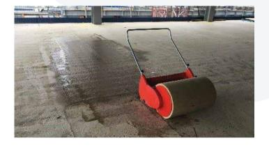
The project Site Manager was attending a sporting fixture and observed a Bowdry machine in use. The water removing roller quickly absorbs excess water and gave a match-ready surface. He realised that the Bowdry was the answer to their water pooling issues he was facing onsite.
